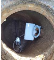
The system operation is supported by rechargeable battery with duration more than 2 months of continuous operation.
